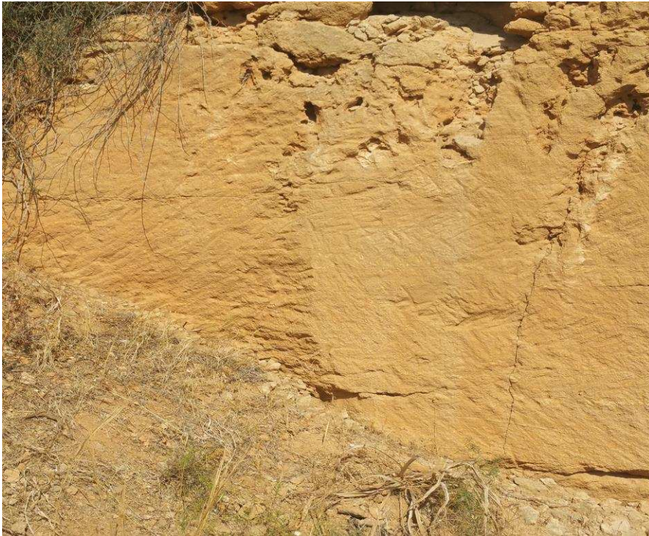
Figure 88: Roman quarry face with chevron-shaped stonemason tool marks evident, sandstone quarry in Paphos in Cyprus.
